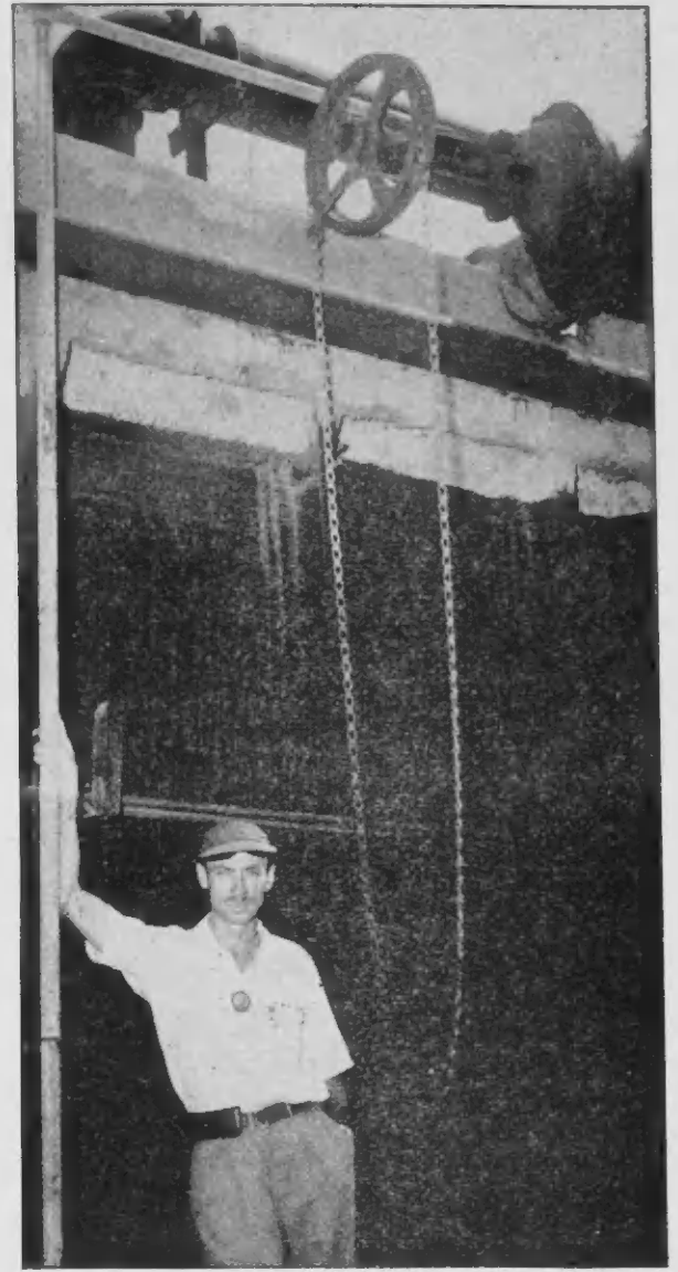
Top CYI Capital Award winner Hendrik van den Arend is shown at left with the suggestion that has earned him Fls. 1750, with an initial of Fls. 750 and the first capital of Fls. 1000. The idea: fresh catalyst must be transferred once a day from the Cat Plant hopper, No. 1, to the loading line, No. 3. Formerly the valve at No. 2 was used, loading through a six-inch line. Mr. van den Arend proposed loading through a small pipe (No. 4) with pressure from the air line, No. 5, with better control and less upset to the operation of the unit.
